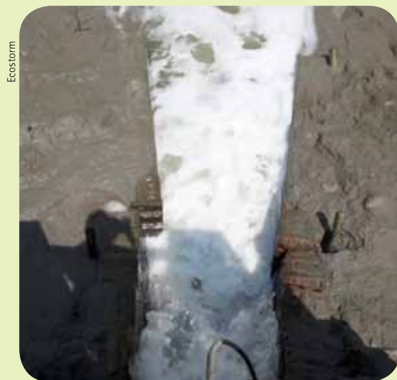
Sluice gates regulate irrigation and flooding of the land.
